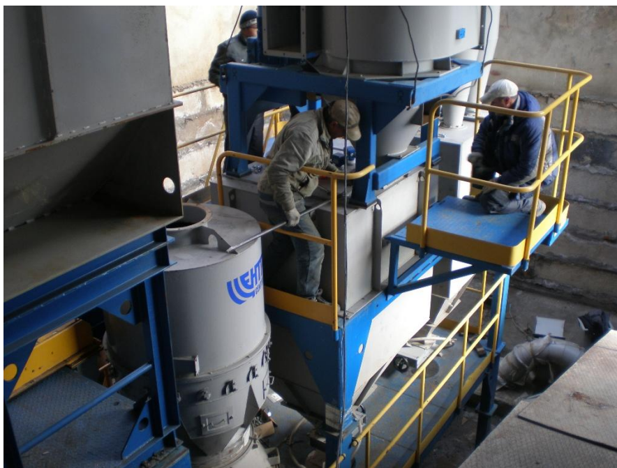
Installation of the technological equipment of CJSC “Ural-Omega”, complex КИ-0,63
